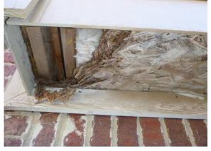
[X] small hole and gap should be sealed beneath the kitchen nook window seat.
