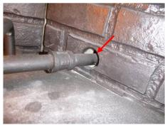
[X] Improper combustion make-up air vent at the exterior of the chimney. This should be a screened opening with a hood to prevent rain intrusion. Purpose is that it helps draw air into a tightly sealed home when the fireplace is on.
