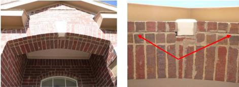
[X] Exterior Missing weep holes over steel lintels above windows, doors, garage door(s) where there is masonry above [IRC code effective 2003].
