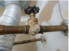
[X] Temperature pressure relief valve (TPR) frozen did not operate. Although the TPR valve may open, I do not force it since the valve may not reseal once opened.
